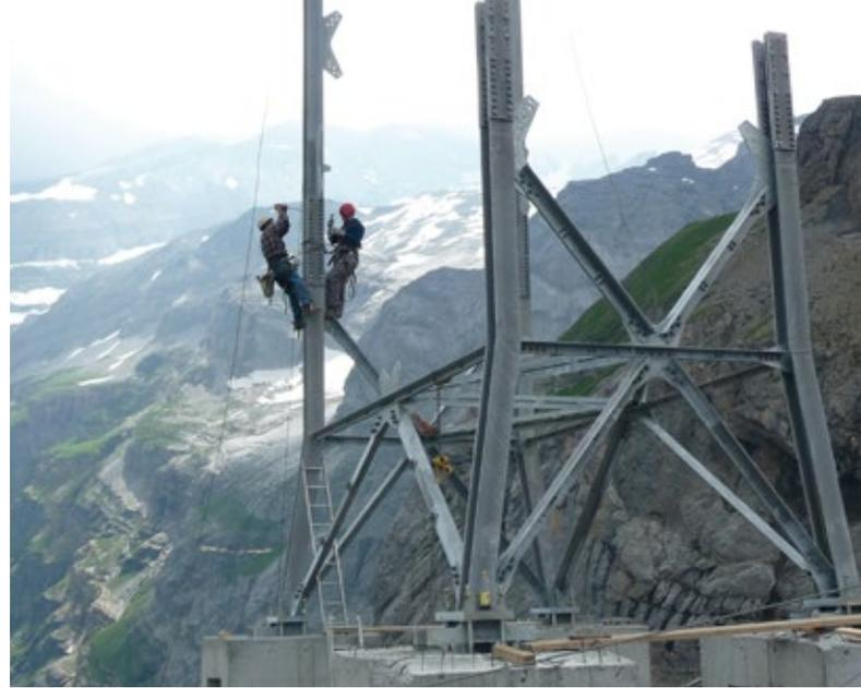
The Garaventa AG is a specialist for cable cars and ropeways. The image above shows the construction of a support structure for the "Linthal 2015" project in Switzerland. (Image: Garaventa AG)
